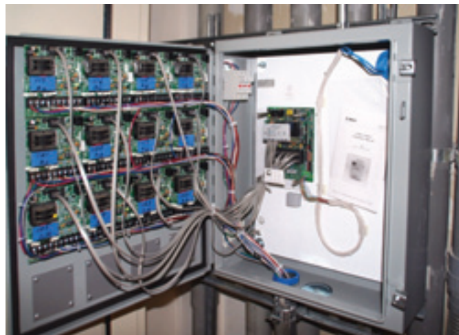
Figure 2. Installable in any convenient location, electric submeters are commercially available in a variety of configurations from single, stand-alone devices to multiple-meter units (shown) housing up to two dozen meters. Applications include benchmarking, measuring and verifying energy conservation and ROI goals in connection with existing building retrofit initiatives gaining momentum around the country.
