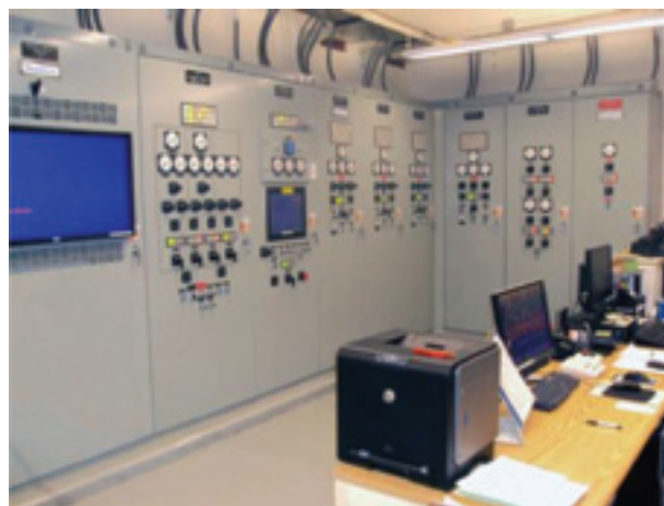
One of two panel boards in the control room at the hospital's power plant. The boards include a custom SCADA system that allows remote monitoring and control of all aspects of the hospital's power system and provides extensive information for analysis and planning. Operators normally access the system through desktop workstations.
