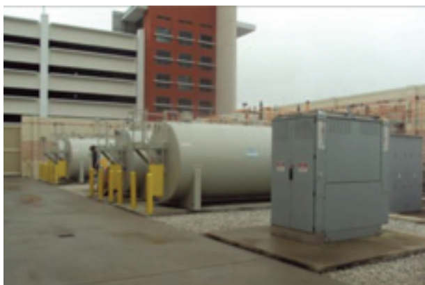
With full tanks, the hospital has enough fuel for 120 hours of backup power if utility feeds are lost. The 2-MW load bank in the foreground facilitates testing of generators.
