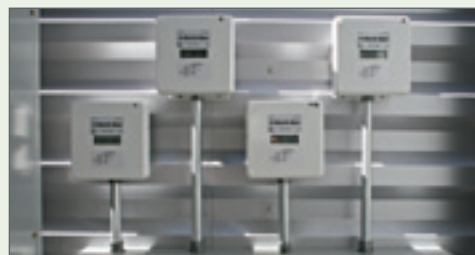
Figure 2: Four 277/480V submeters were installed next to a main switchgear cabinet outside one of the buildings.
